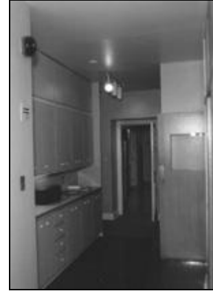
There is a major circulation problem at the servery.
