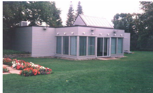
Pool Building (photo NCC 1998)
