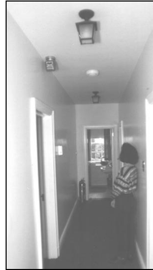
In case of outage there is only minimal battery pack lighting.
