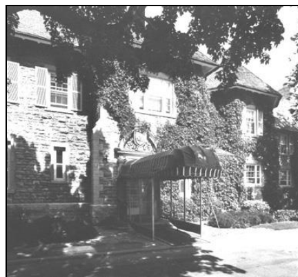
A suitable winter enclosure is needed at front entrance.
