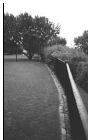
Rebuild the fence at the top of the escarpment.
