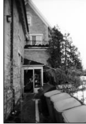
Inadequate screening for garbage containers
