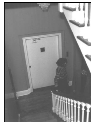
Elevator door opens into stair
