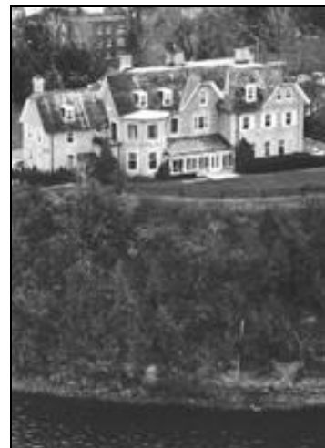
Escarpment is prone to erosion.
